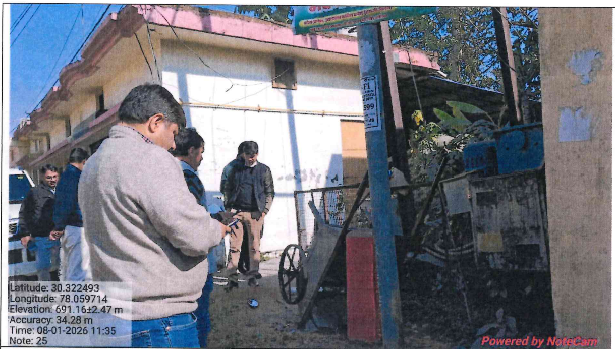
Site 2 : Government : Transformer room
